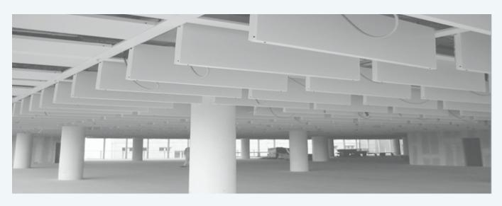
The radiant panel heating and cooling systems of S&L are equipped with a new highly integrative installation concept, which provides markedly efficient and eco-friendly operations. Suitable for a variety of heating and climate requirements for floor, ceiling or wall installation, the systems work completely draught-free. Both heating and cooling is provided by just one pipe system. Since
