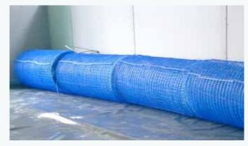
The flexible capillary tube mats are connected by socket welding to each other and to the pipeline network. Main collectors and pipelines are laid in the recess of the previously installed heat and sound impact insulation. The capillary tube mats continue to be rolled up. Then, the PP-Floor capillary tube system
