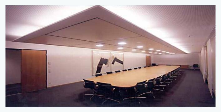
This is a heating and cooling ceiling. As a closed radiation ceiling it is used for on site installation of smooth or perforated metal ceilings. As a closed air conditioning ceiling, it dissipates sensible thermal loads of about 60% by radiation and of about 40% by convection.
