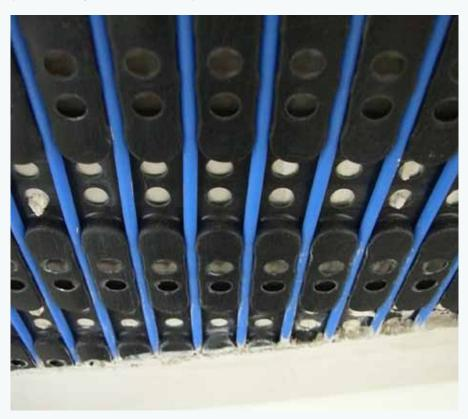
mats) is bonded to the firm and dry surface with filler substance. Afterwards, the mats are installed on the ceiling while applying adhesive filler substance with a toothed trowel with a tooth size of
