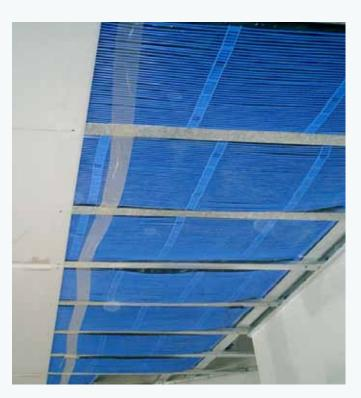
To ensure that the required even pressure loss is guaranteed within the mat surface, the capillary tubes have a low permeability. Moreover, because of the reduced crystallinity of an extraction-stable polymer, a high flexibility is also given at low operating temperatures. The capillary tube mats are fastened with open welding ends to the already
