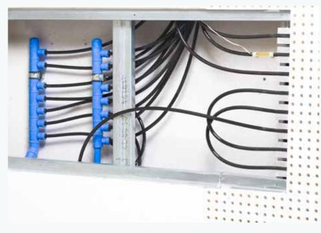
pipe installation, with the necessary pipe distance intervals of around 50 mm. The maximum tube length per register element is up to 50 m; the tube length difference between registers within a heating-cooling circuit including connections for the air-conditioning water is about 15%. Due to the possible on site installation, the system is especially characterised by its high flexibility. Within the ceiling voids, the connections of the air condi-
