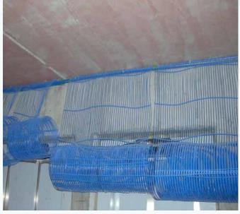
This system consists of mat modules. These are made of parallel guided capillary tubes that are incorporated homogenously into the oval distributor/collector. Furthermore, they have a modular form with mutual welded quick fasteners (plug-in system) for a connection to the supply and return line by means of two pieces of flexible tubes. Because
